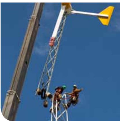
Construction complete in less than two weeks
