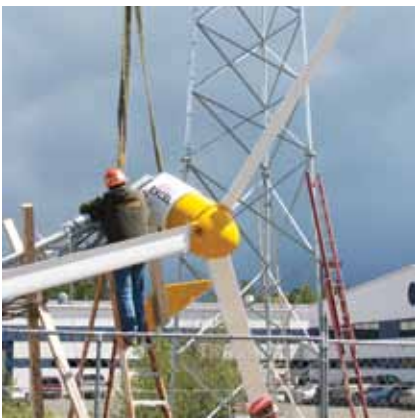
Experienced Alpha installers
