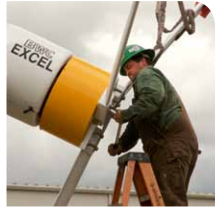
7.5kW wind turbine generates energy in winds as little as 8MPH
