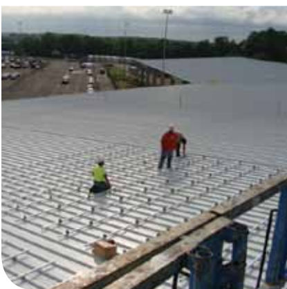
Required 8,000 hold down clamps
