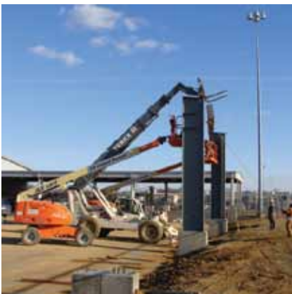
Solar panels weighed approximately 220,000 pounds
