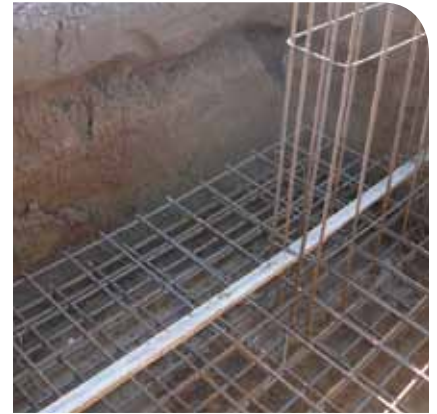
Required 240 cubic yards of concrete
