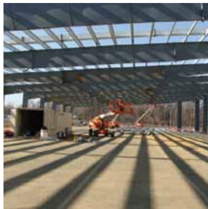
More than 550,000 pounds of steel
