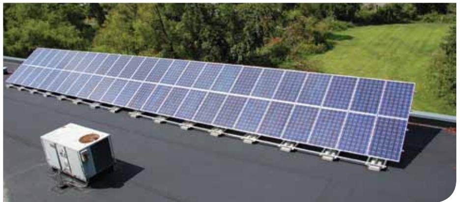
Completed array of 48 panels that provide 11.28kW DC power
