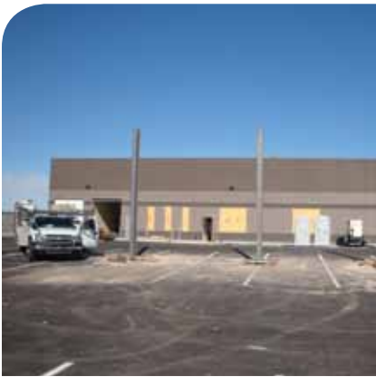
Open parking space dedicated to solar power
