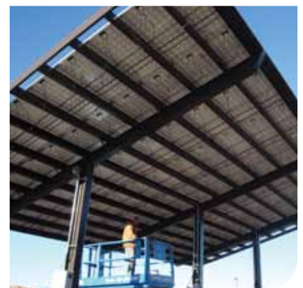
Created 12 covered parking spaces
