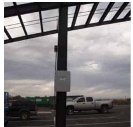
Required three 600kW inverters
