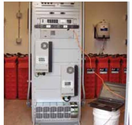
Hybrid system includes a 20kW diesel generator and 48VDC battery bank
