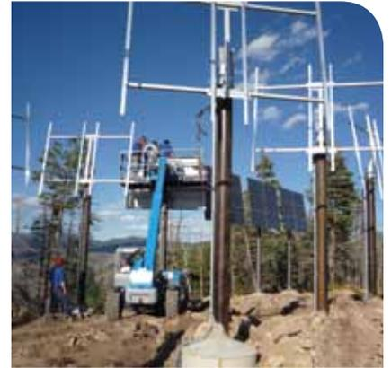
Custom engineered to withstand 125MPH wind load
